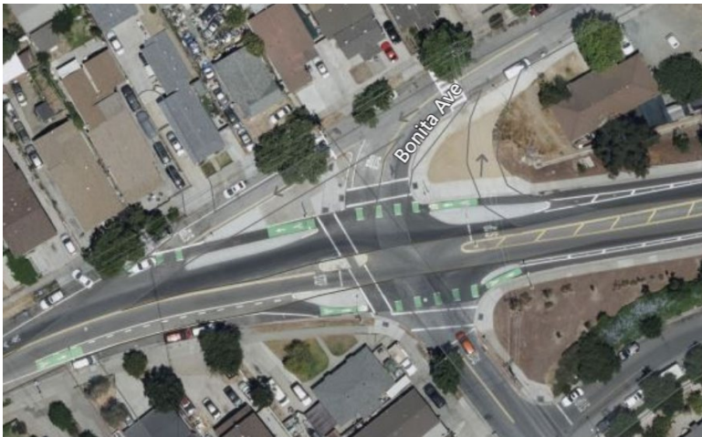
6 - Protected intersection at San Antonio St and Bonita Ave
