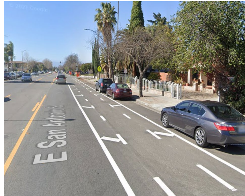
9 - Buffered bike lanes on San Antonio St
