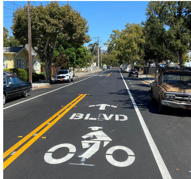
4 - Bike boulevard roadway markings on St. John St
