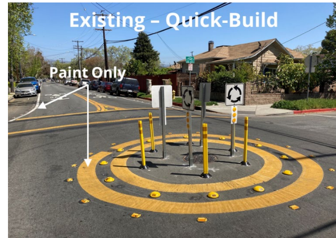
29 - Existing quick-build traffic circle
