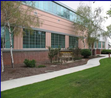
Central Service Yard
