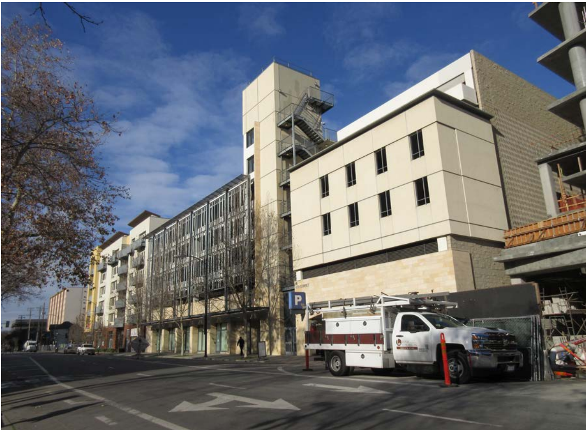
Photo 4: View of the surrounding development looking northeast from North Fourth Street.
