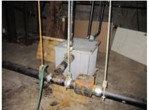
Photograph 4. Grease trap in basement.
