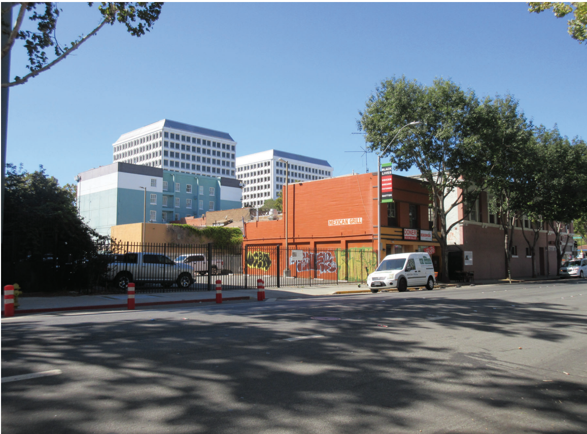
Photo 3: View of project site and surrounding development, looking northwest on South Fourth Street.
