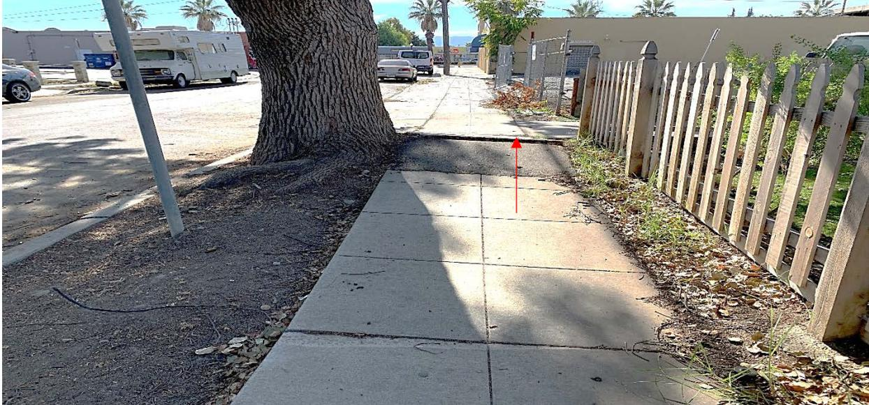
**Image #10 – Tree T95. Sidewalk has been lifted by diameter expansion of buttress roots. Repairs have been made, but a 2-inch grade difference at asphalt to concrete seam creates a trip hazard (arrow).**
