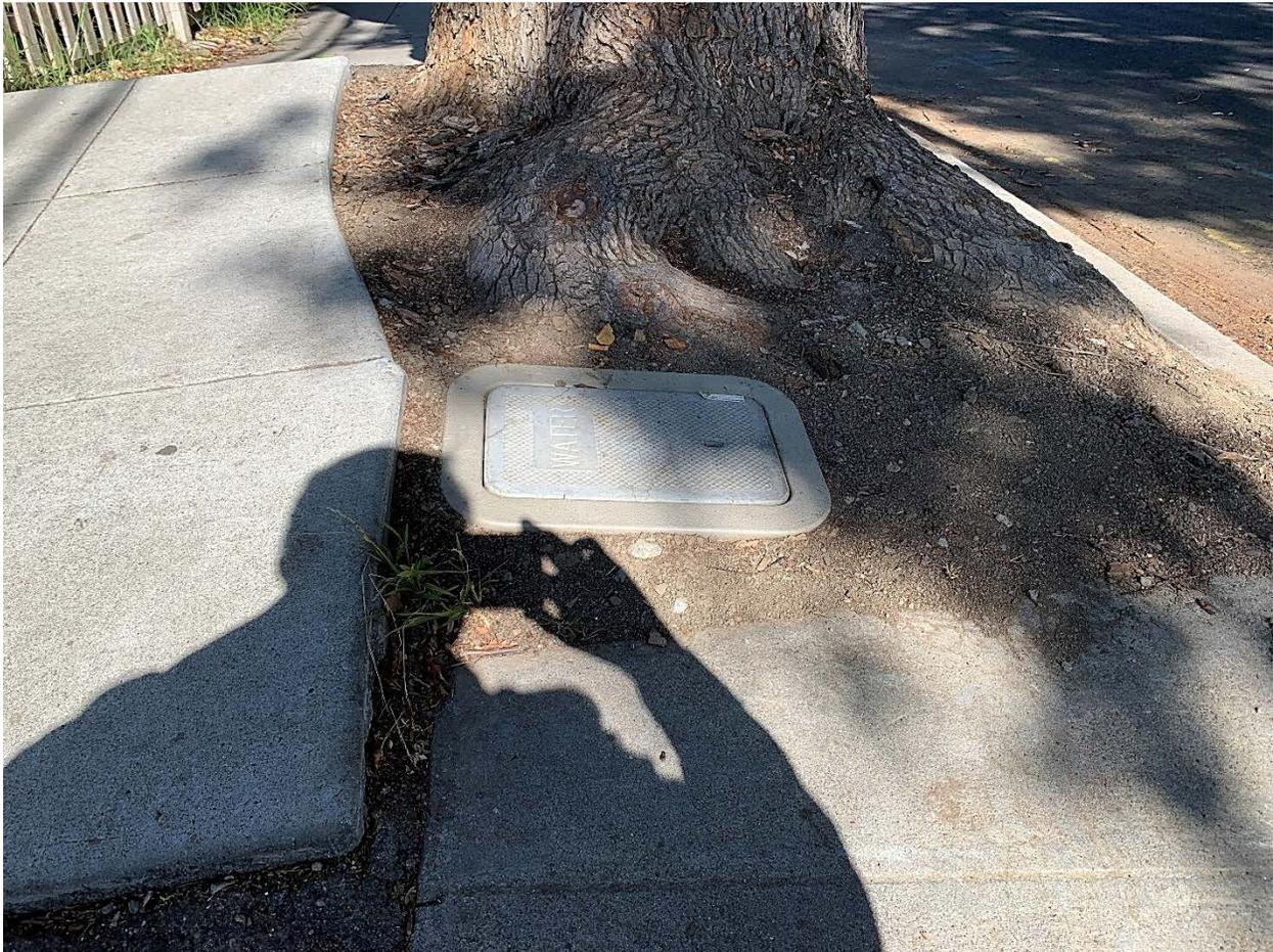
**Image # 11, Tree T95, camphor. The remaining space for the water meter box and utility line will decrease over time. Note lifted sidewalk.**
