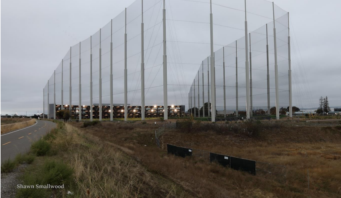
Photos 15 and 16. Depiction of the TopGolf site's illumination at night, according to the IS/MND prepared for the TopGolf project (top), and the actual type of illumination visible on the morning of 30 October 2021 (bottom). The lights on the building were sufficiently powerful to illuminate the poles supporting the net at the southern end of the project, and when I first arrived, the site of the proposed project was also lit by the TopGolf project. The lights appeared much brighter than could be shown in a photo. Note also that the moon would never occur where the IS/MND depicted it, which was north of the project.
