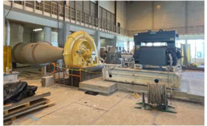
New motor installed on Secondary Blower #2
