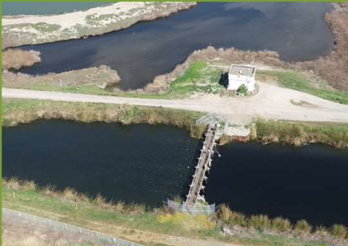
The weir structure and Sulfur Dioxide building at the outfall channel.
