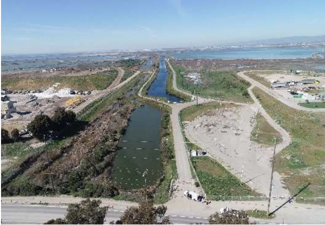
January 2022 aerial view of the Outfall Channel and Instrumentation Improvements Project.
