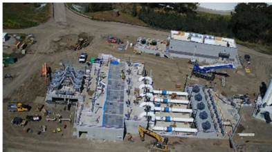
Aerial view of the new Raw Sewage Pump Station and Grit Facility.
