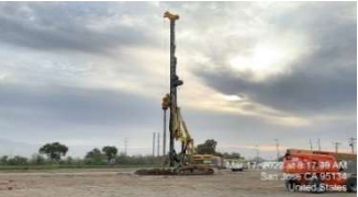
Stone columns being installed for the new dewatering facility.
