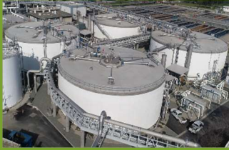
Aerial View of the Digesters
