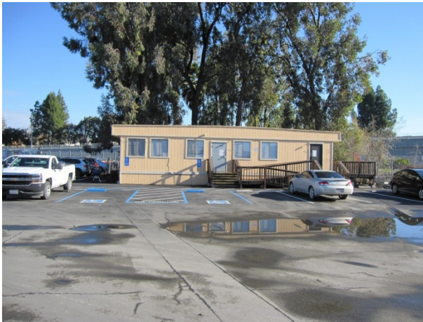
Photograph 3. Office building occupied by AT&T, looking east.
