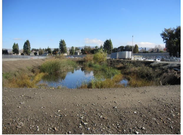
Photograph 2. On-Site storm water retention basin, looking east.
