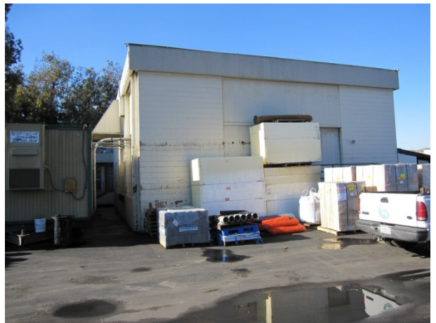
Photograph 10. Warehouse building occupied by Maniglia Landscape, looking west.
