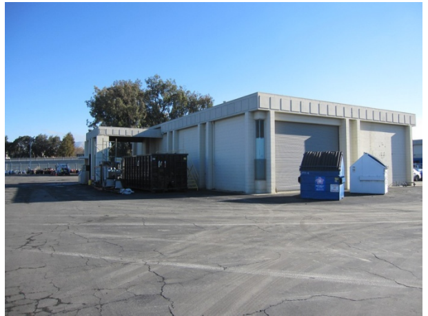
Photograph 4. Warehouse building occupied by AT&T, looking east.
