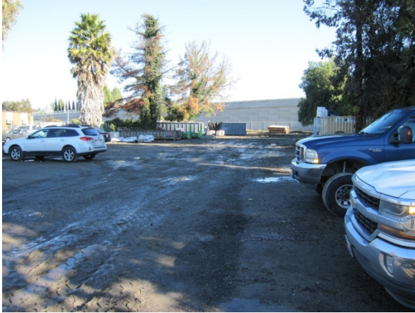
Photograph 13. Construction staging and parking area used by Western National Builders.
