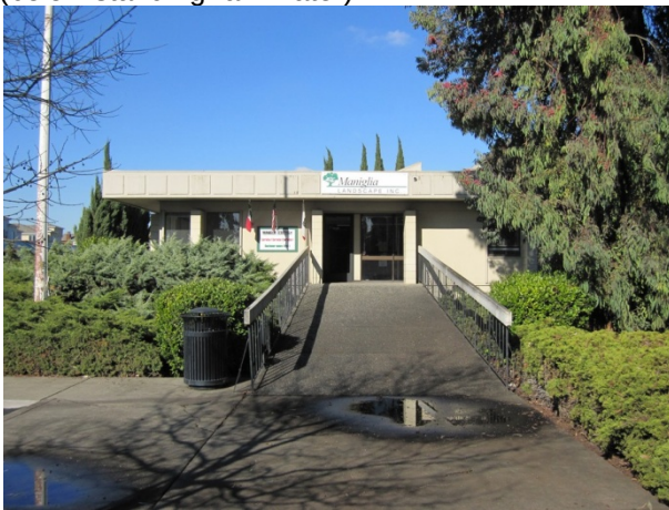
Photograph 9. Office building occupied by Maniglia Landscape, looking north.
