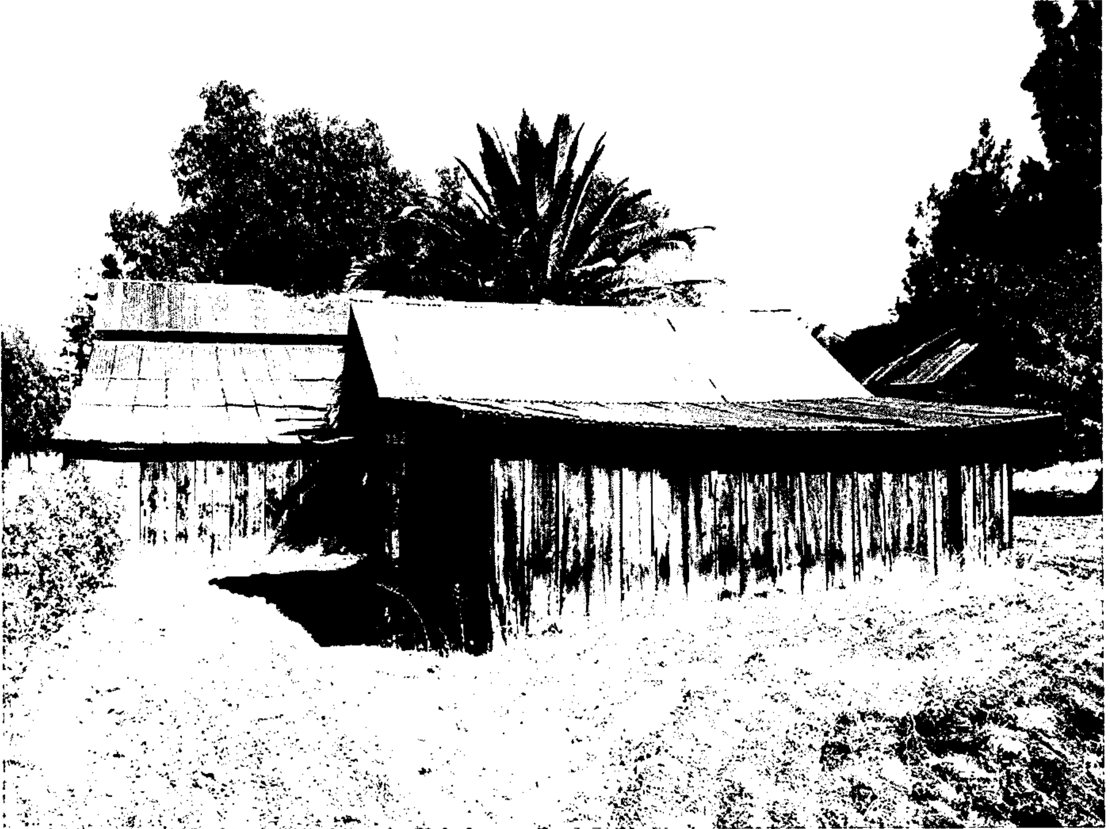
2740 Ruby Avenue- Ancillary agricultural buildings View; the barns and garages are grouped in the center of the property. Camera facing North Date October 13, 2015
