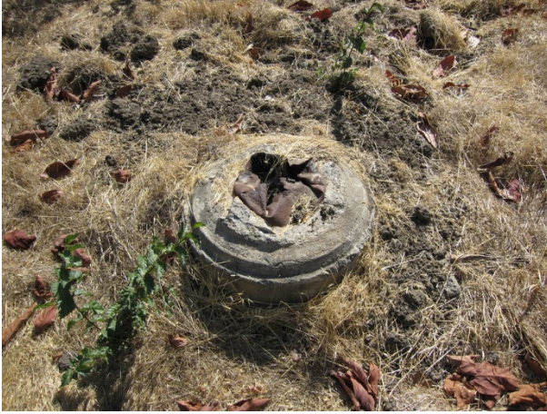
Photograph 5. Water supply well.
