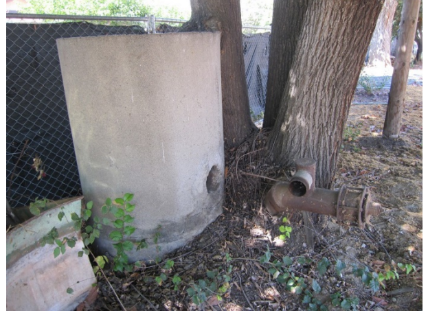
Photograph 6. Apparent standpipe and irrigation piping.
