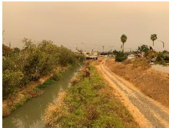
Looking downstream at the McKee Road culvert
