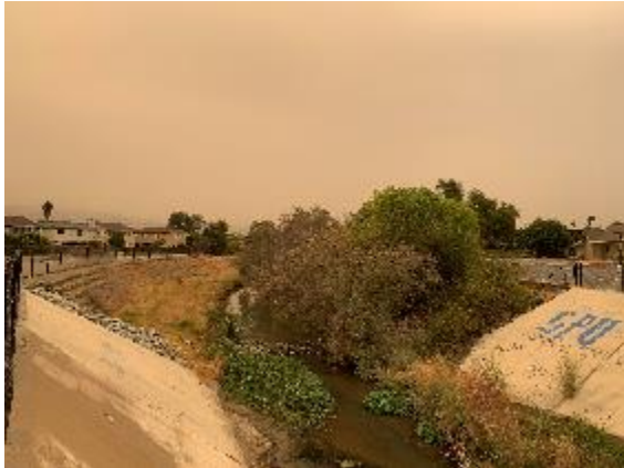
Looking upstream from San Antonio Road
