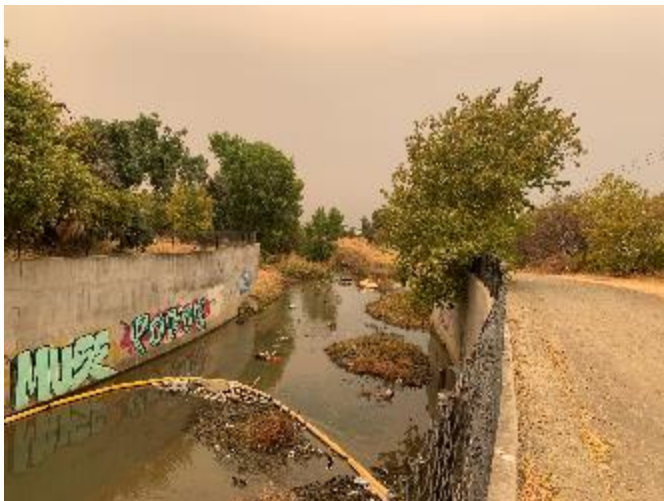
Looking downstream from the upstream end of Reach 1
