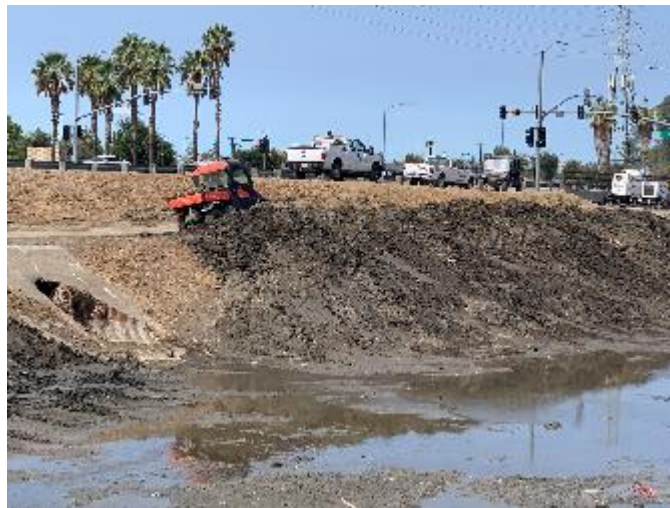
Beginning of Reach 8 at Confluence with Thompson
