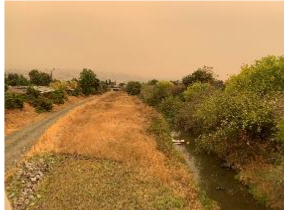
Looking upstream from Kammerer Pedestrian bridge towards I-680
