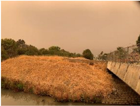
Looking west down floodwall and levee at Cunningham Avenue (culvert on right)
