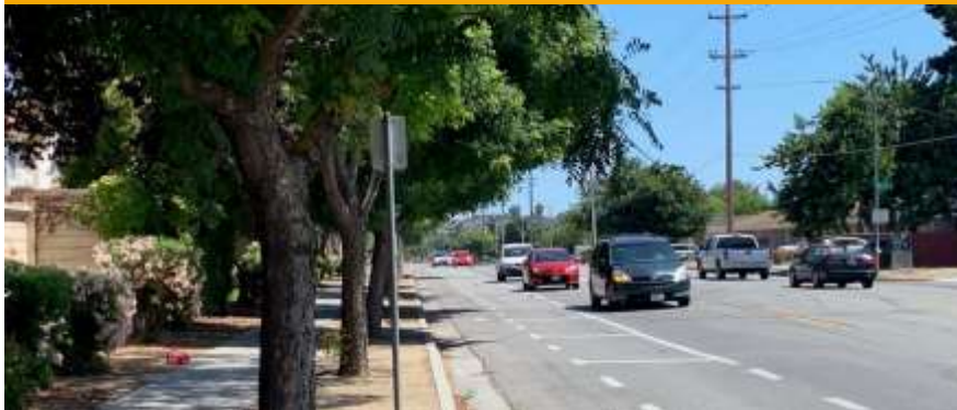
Wide roadway encouraging high speed
