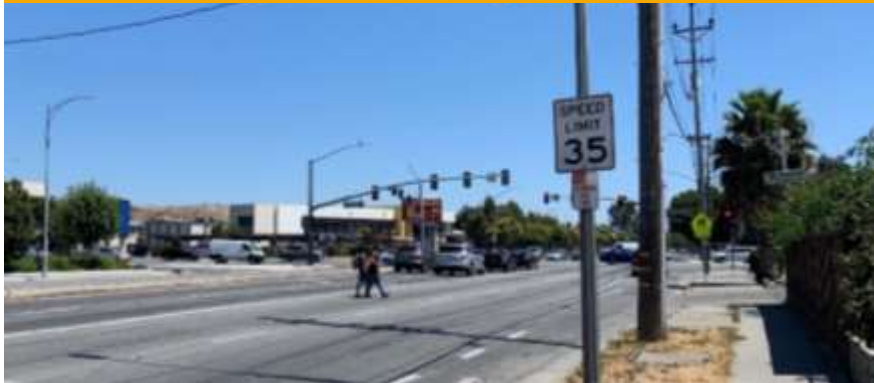
Long distances between marked crossings
