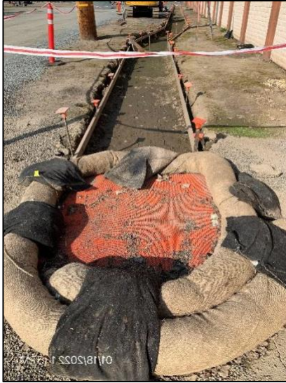
Effective BMPs installed at construction site.
