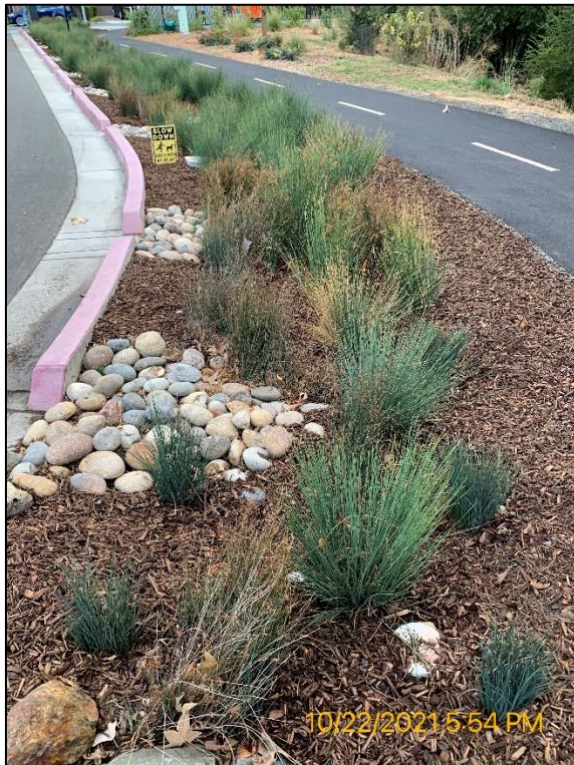
Bioretention Area along the Guadalupe Mines Trail.
