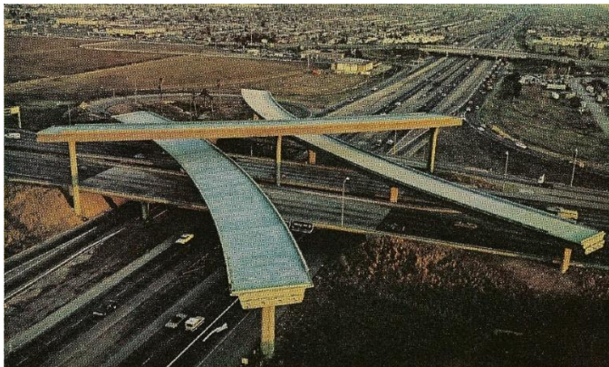
Figure 10: The 680, 280, and 101 freeway interchange, under construction in 1976
