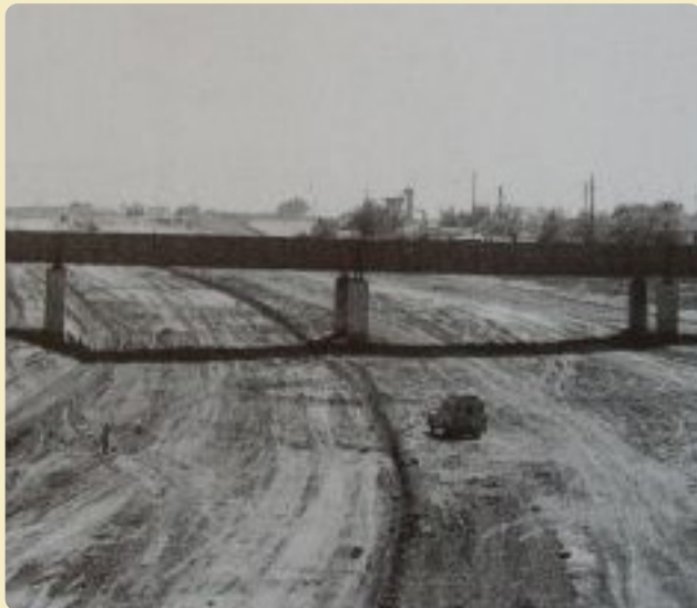
I-280 CONSTRUCTION, 1970 - SOUTH UNIVERSITY NEIGHBORHOOD
