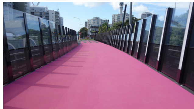
NELSON STREET CYCLEWAY IN AUCKLAND NEW ZEALAND.
