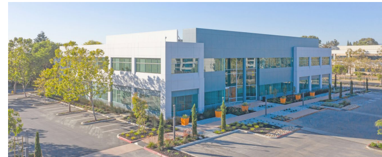
Low-Rise Commercial Office
