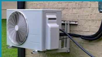
**Ductless mini-splits** are decentralized heating and cooling systems that allow the user to control the temperatures in individual rooms or spaces. Mini-split systems have two main components -- an outdoor compressor/condenser and an indoor air-handling unit(s). The mini-split transfers heat between a house and the outside air via refrigerant lines, not requiring the use of ducts.
