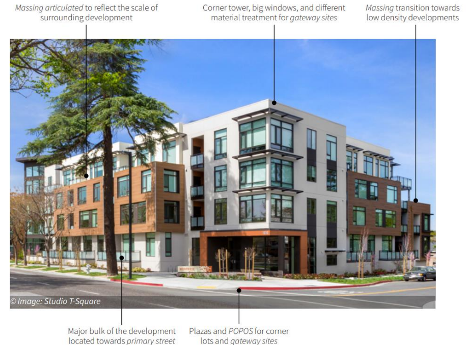
Fig. 3.1 Locate activities to complement existing nearby uses, design buildings to follow prevailing setbacks, and articulate building massing to match the scale of adjacent developments.
