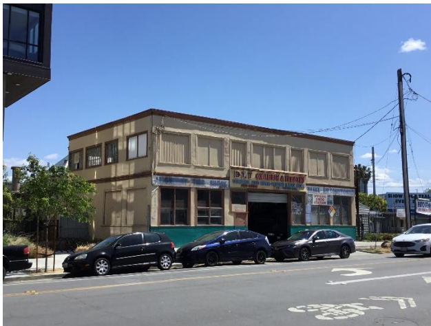
Northwest and Southwest elevations, viewing East.
