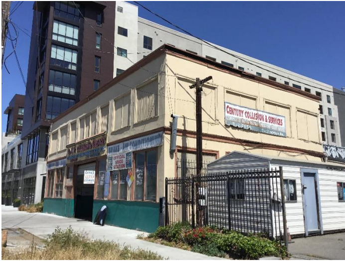
Figure 2. 60 Stockton Avenue, southwest and southeast elevations, view north.
