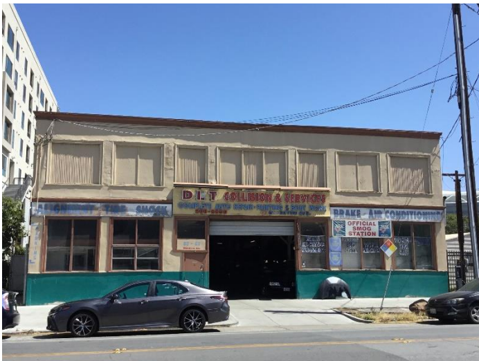
Figure 3. 60 Stockton Avenue, frontage view, southwest elevation, view northeast.
