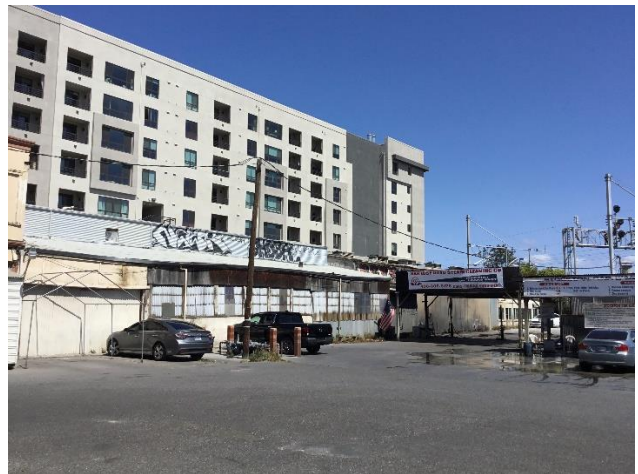
Northern portion of Southeast elevation, viewing North.
