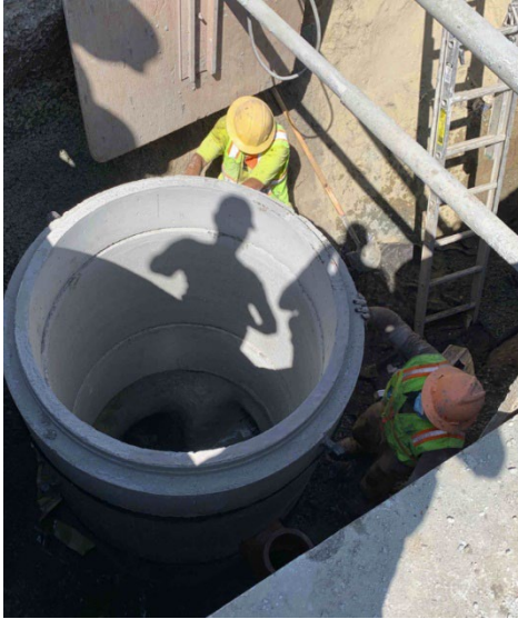
Sierra Road Sanitary Sewer Improvements (Manhole Installation)
