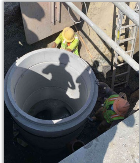
Sierra Road Sanitary Sewer Improvement (manhole installation)
