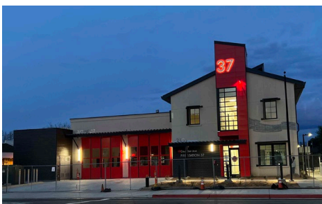
Completion of Fire Station 37
