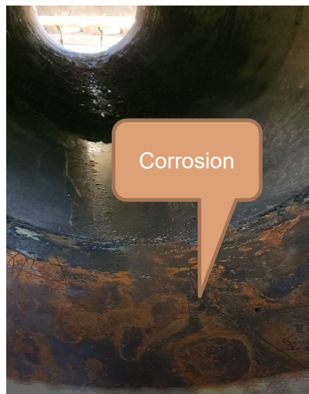
Pipe Corrosion
