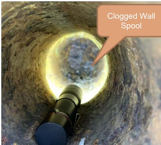
Groundwater Relief Valve Wall Spool
