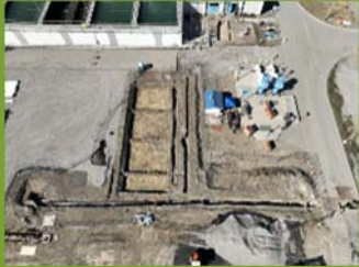
Excavation for electrical duct banks near the Filtration Building.
