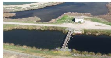
The weir structure and Sulfur Dioxide building at the outfall channel.
