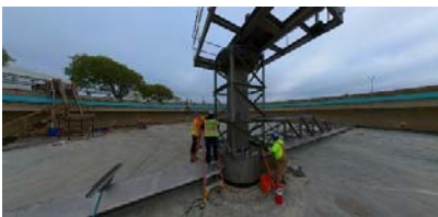
Contractor assembling the clarifier mechanism at nitrification clarifier B6.
