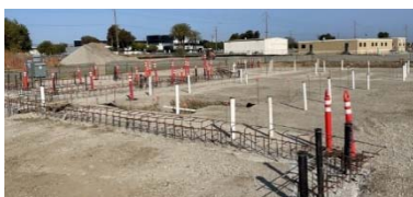
Dewatering Building Sewer and Process Drain pipe.
