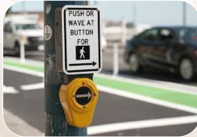
Accessible Pedestrian Signals (APS)
