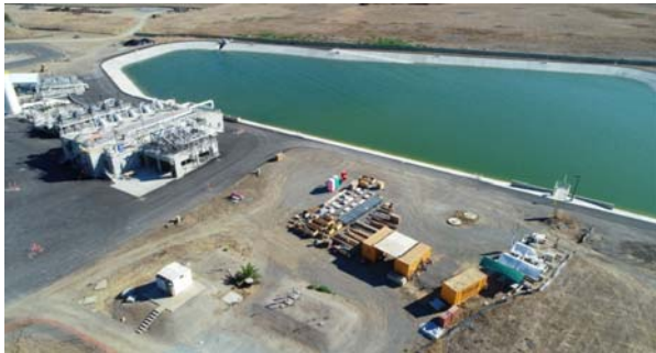
September 2022 aerial view of the Emergency Overflow Basin of Headworks Project.
