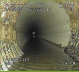
CCTV of Storm Drain
