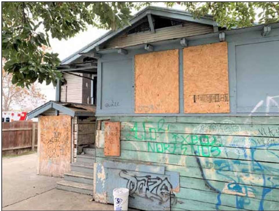
Photograph 5: Detail view of rear addition; facing southeast, January 18, 2022.
