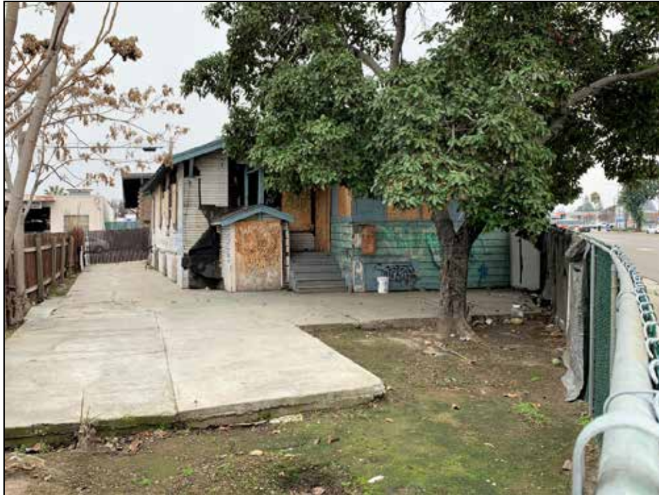
Photograph 4: Rear north side of residence; facing south, January 18, 2022.
