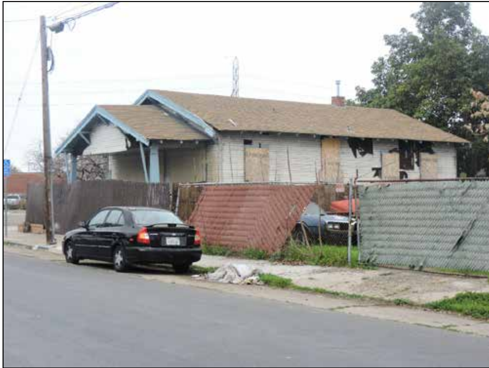
Photograph 2: South façade and east elevation; facing northwest, January 18, 2022.
