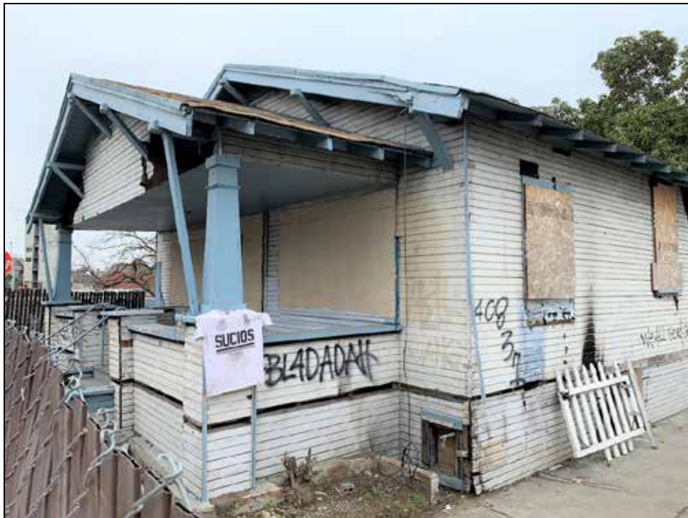
Photograph 3: Front porch detail; facing northwest, January 18, 2022.
