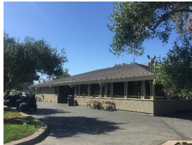
Clubhouse and Patio
