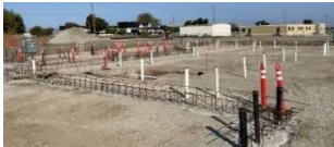
Dewatering Building Sewer and Process Drainpipe.
