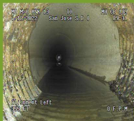
CCTV of Storm Drain
