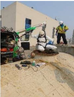
Project Site – Yard Piping Phase 2
