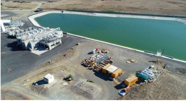
Aerial view of the Emergency Overflow Basin of Headworks Project.
