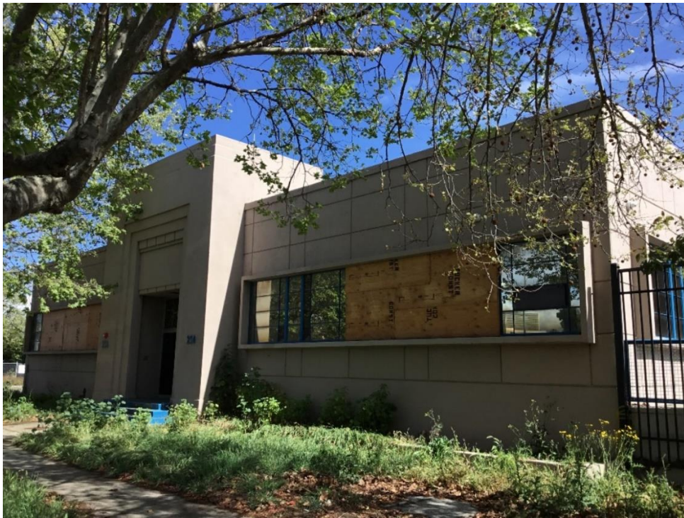
Figure 4. The southwest elevation of 250 Stockton Avenue, view north, March 28, 2022.
