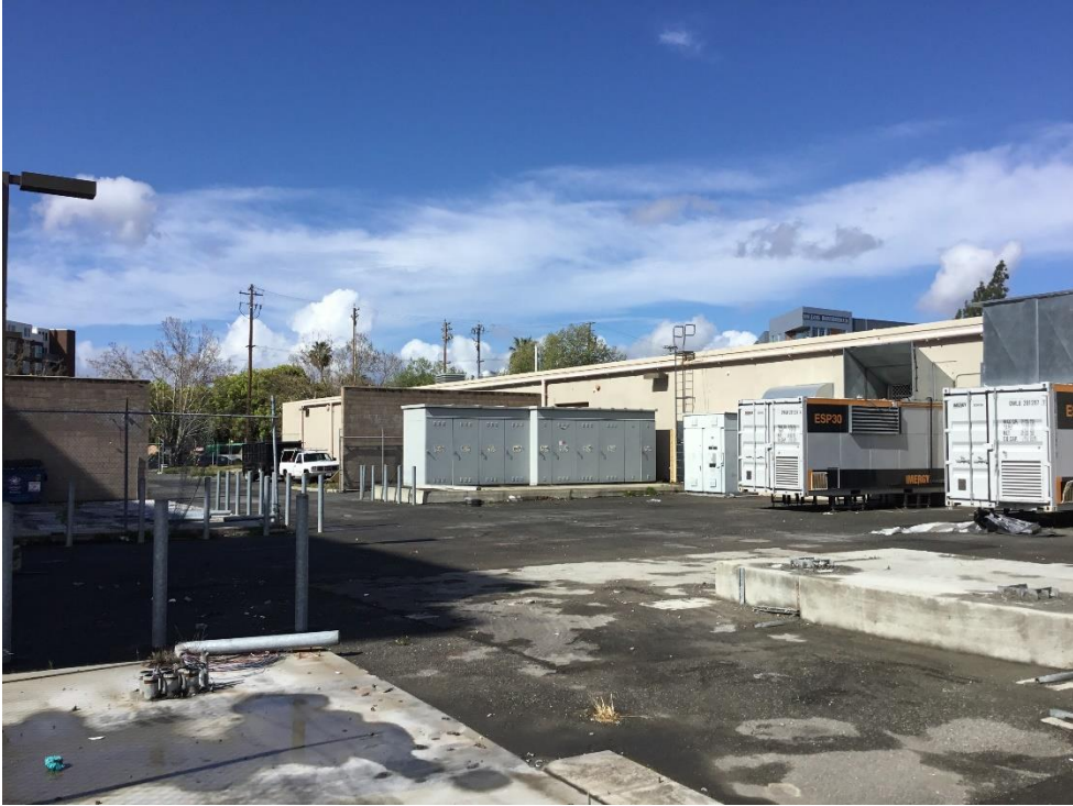
Southeast elevation facing west.
