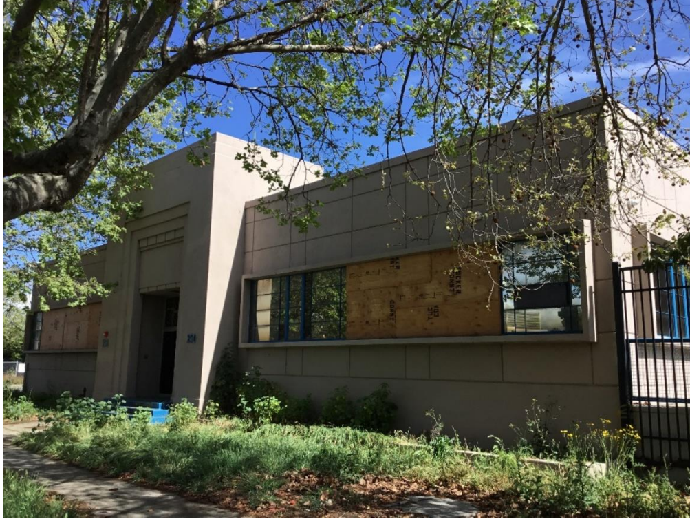
Southwest elevation facing north.
