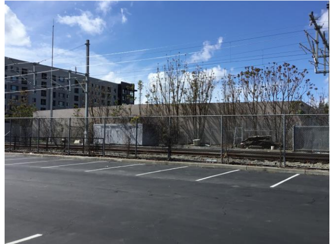
Northeast elevation, viewing South
