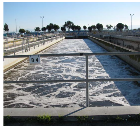
Nitrification tank B-4.
