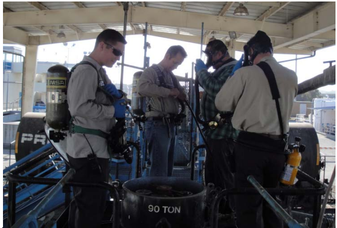
Plant operators prepare to close the dome gas valve on the last chlorine rail car after 40 years of gas disinfection.
