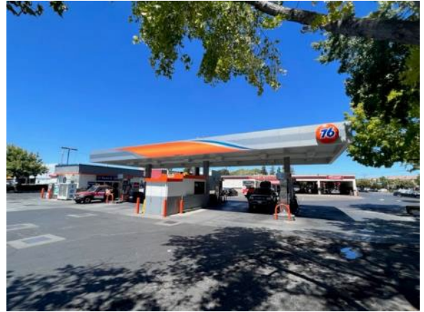
Photograph 7. Building 4 gas station with pump station and canopy. View northwest. August 12, 2022.
