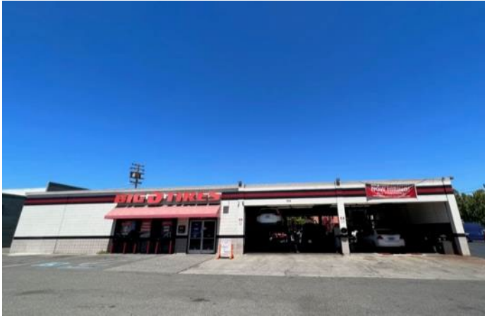
Photograph 6. Building 3 south (main façade). View north. August 12, 2022.
