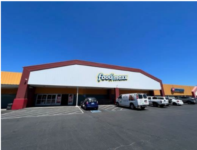
Photograph 2. Central storefront entrance at Building 1. South façade, view northeast. August 12, 2022.
