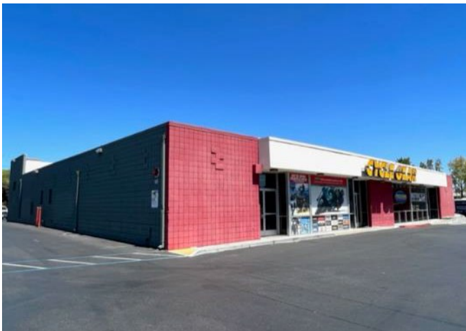
Photograph 4. Building 2 corner view of south (main façade) and west walls. View northeast. August 12, 2022.
