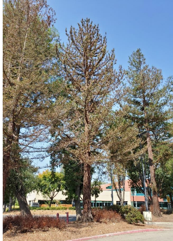
Figure 3. The redwoods (#648 at center) are highly sensitive to salinity and are suffering from recycled water damage. Unless there is a switch back to potable water, the trees would likely not recover.
