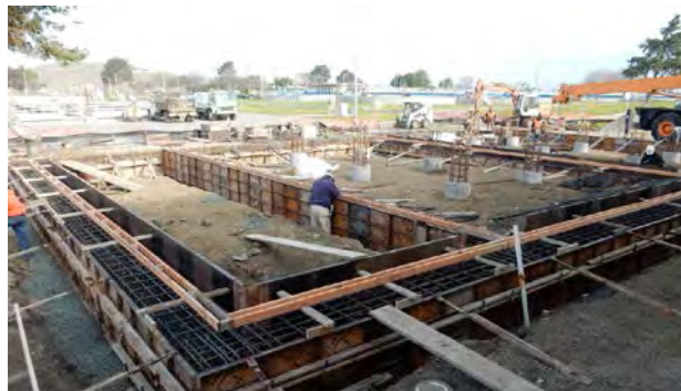
Work in progress on new digester gas compressor building – January 2015
