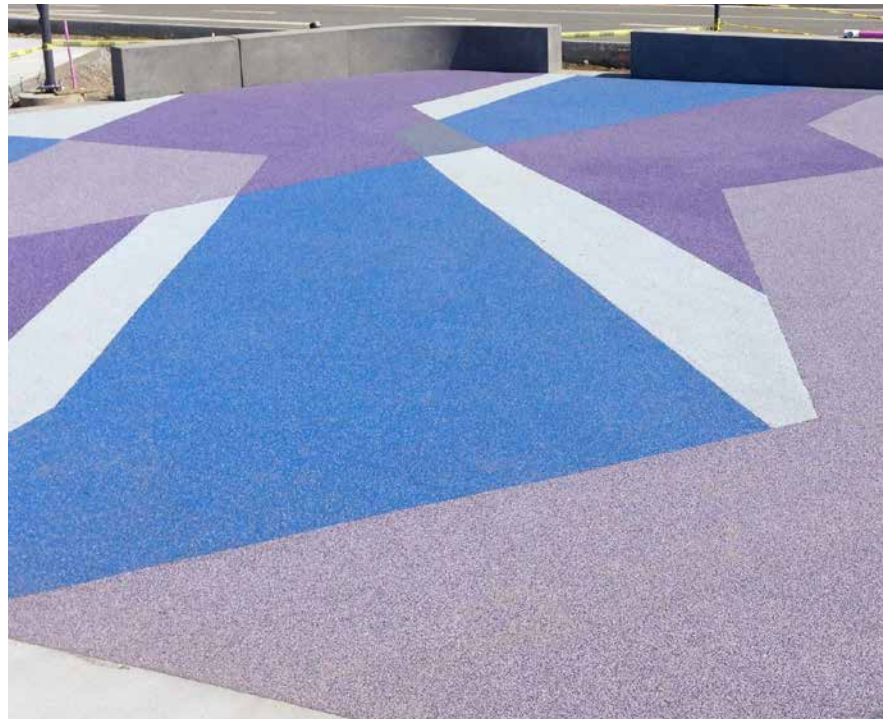
Rubberized Play Surfacing
