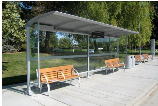
A transit stop with bench seating, shade cover, trash receptacles, and transit information.
