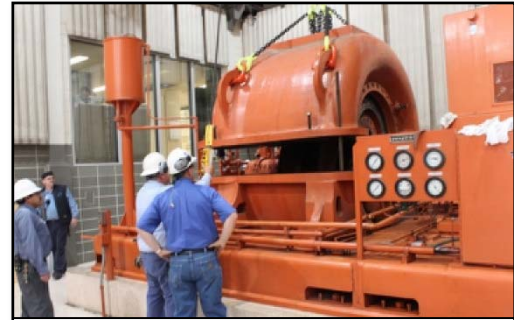
Assessment team inspecting blower TBB-3
