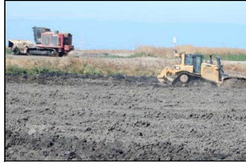
Fecon and Caterpillar tractors at work in biosolids drying beds.
