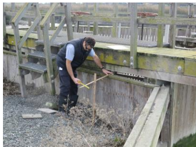
Bryan Frueh checks movement of southern structure.
