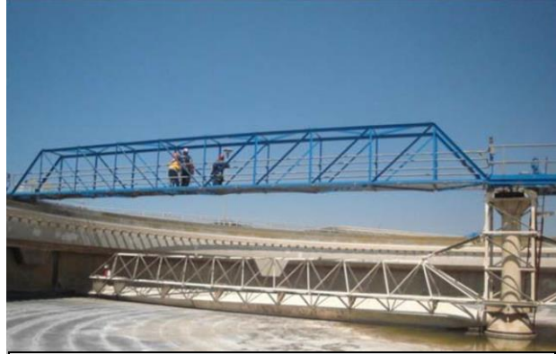
Worker on a clarifier “Tow-Bro” arm.
