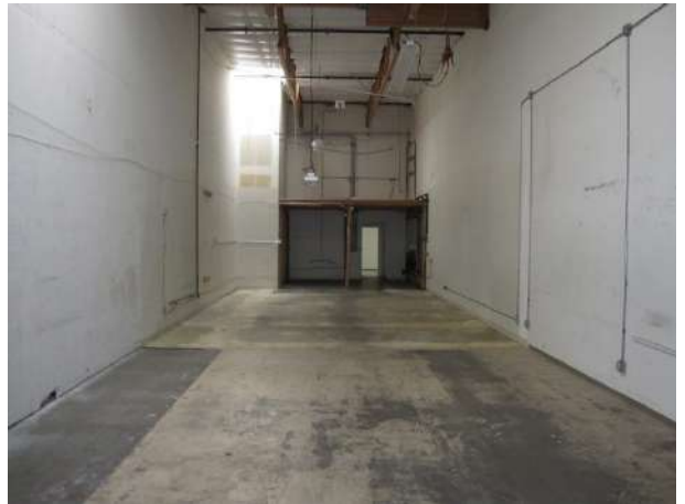
Photograph 4. Unoccupied tenant space.
