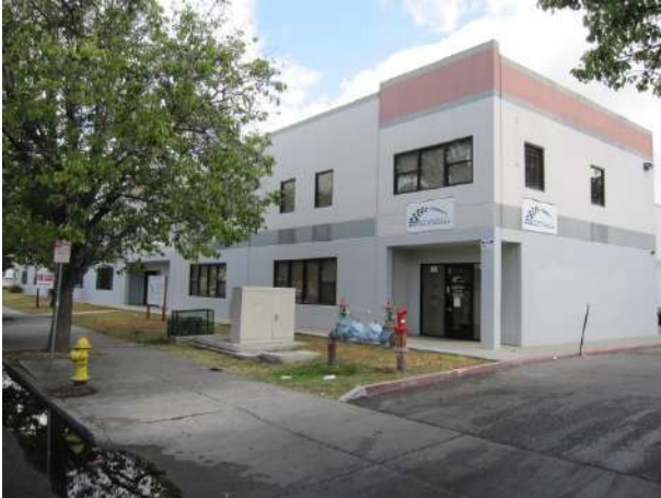
Photograph 1. View of the on-Site building looking north.
