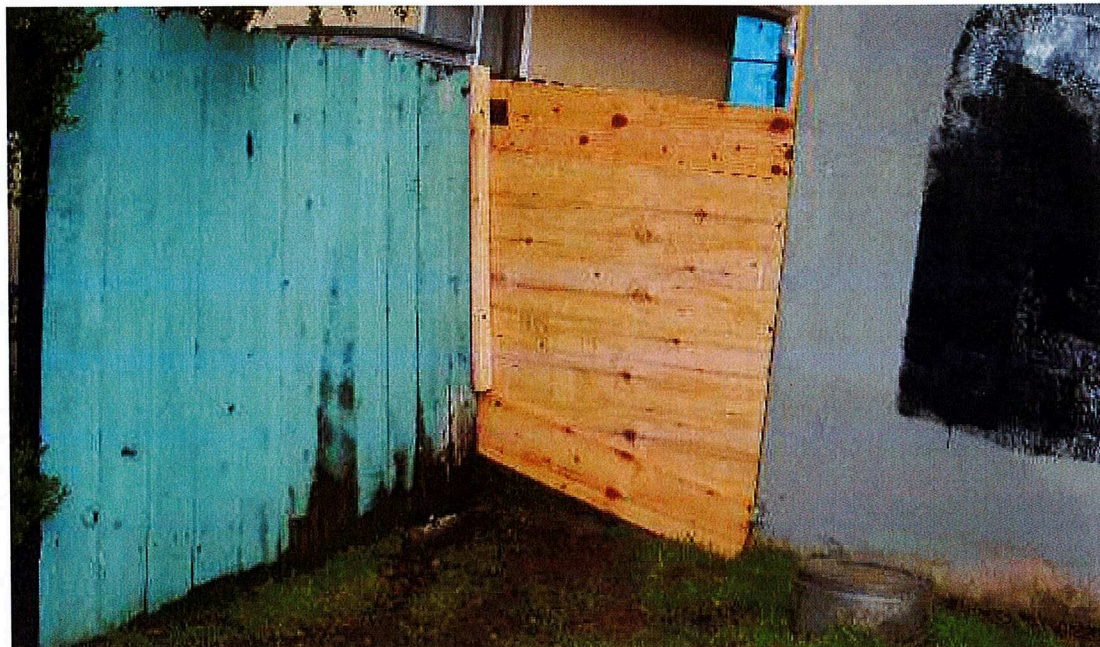
1-28-21 Left side of property secured with plywood fencing
