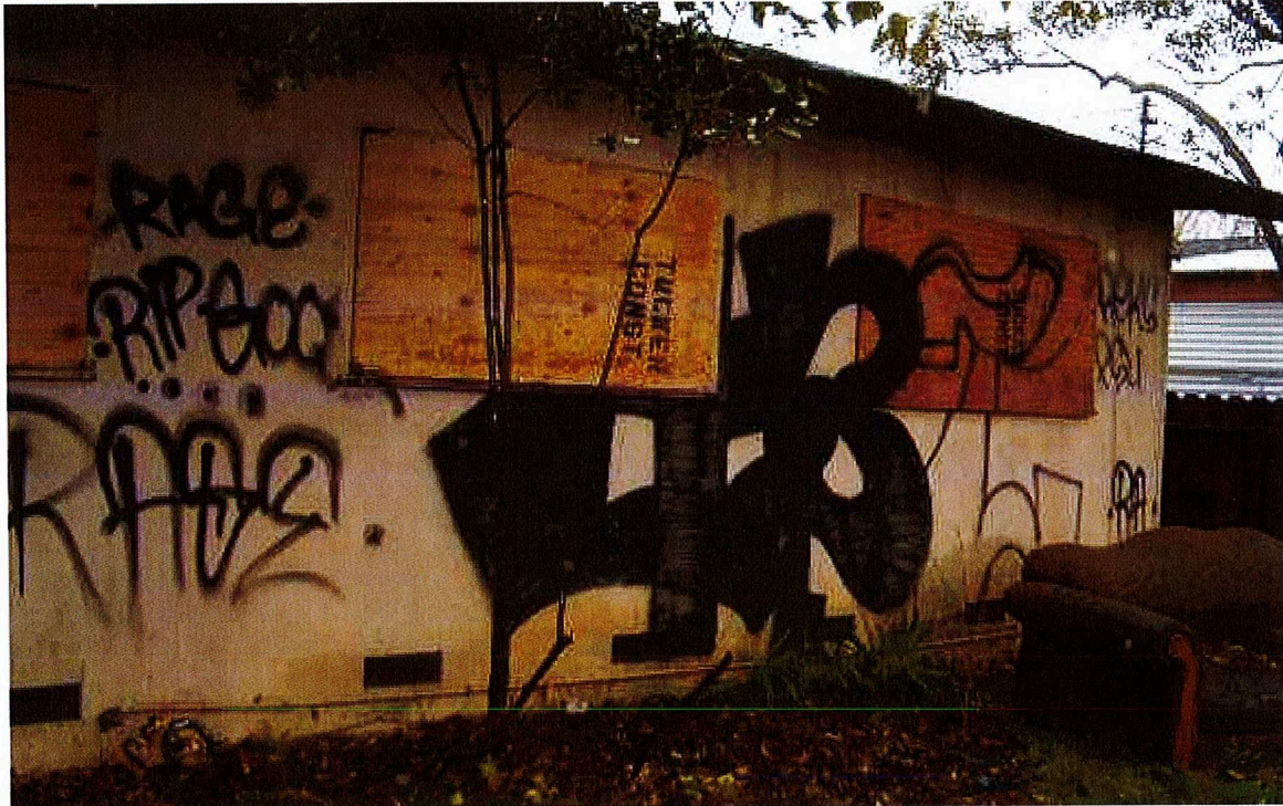
1-28-21 Rear windows secured
