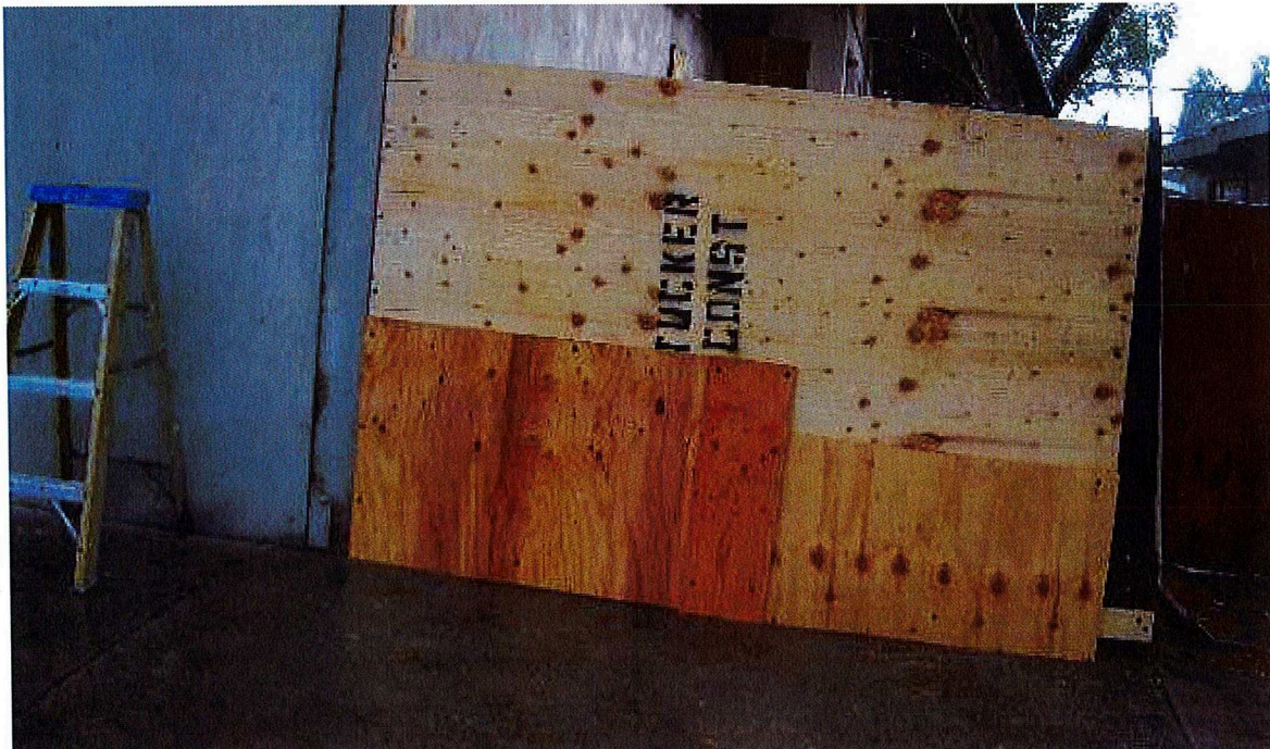
1-28-21 Right side of property secured with plywood fencing
