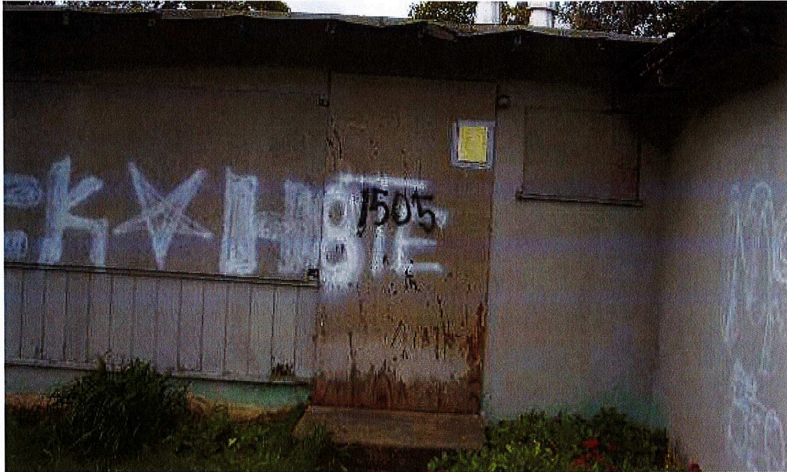
1-26-21 Front door to home with Official Warning notice posted
