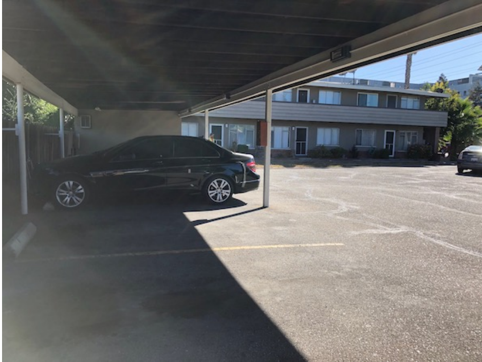
Photograph 6. View looking east-southeast at carport and two-story apartment building in southeast corner of Site.
