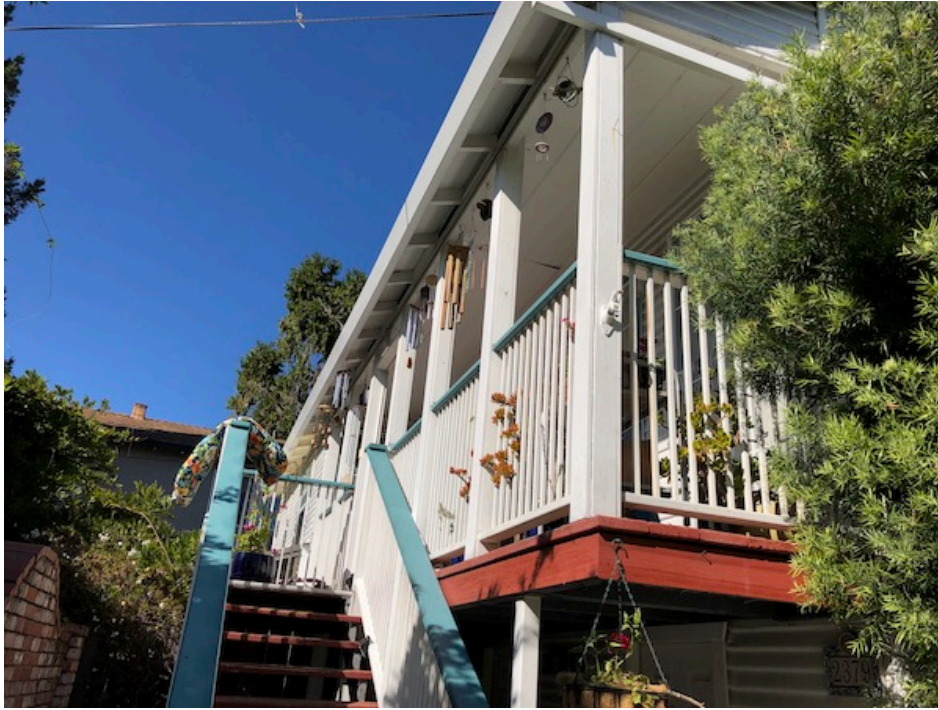
Photograph 38. Second floor of apartment building.
