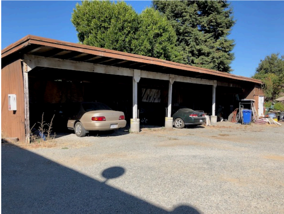
Photograph 22. Carport in northwestern portion of Site.
