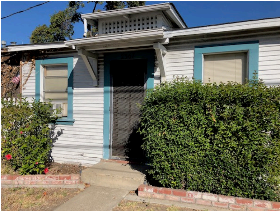
Photograph 15. One of six cottages (parcel with address of 2369 Moorpark) along southern-central portion of Site.
