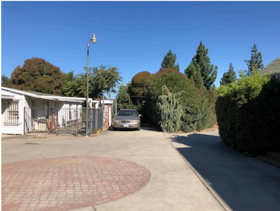
Photograph 43. Alternate view of single-story tenant unit.
