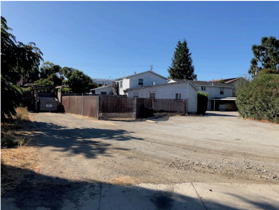
Photograph 3. View looking southwest across vacant lot / driveway access from Central Way.
