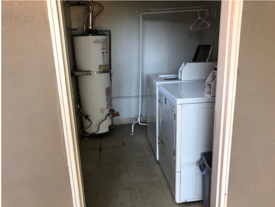
Photograph 8. Laundry room adjacent to carport.
