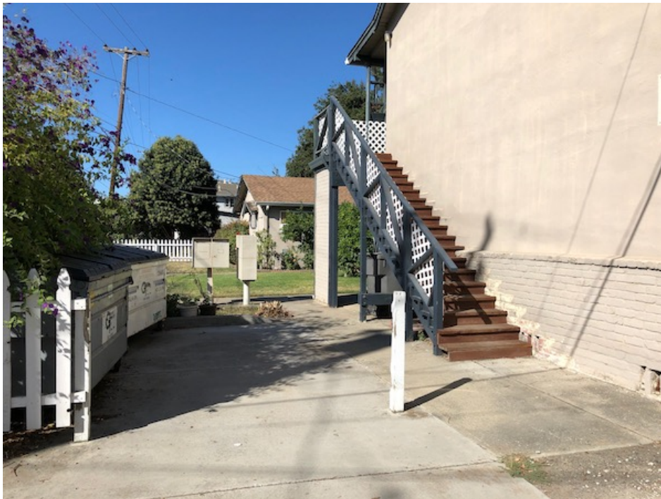
Photograph 31. View looking west along southern side of 2389 Moorpark apartments.
