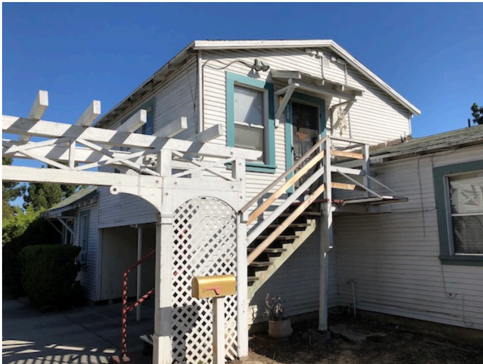
Photograph 39. Another residential structure in north-central portion of Site (2373 Moorpark).
