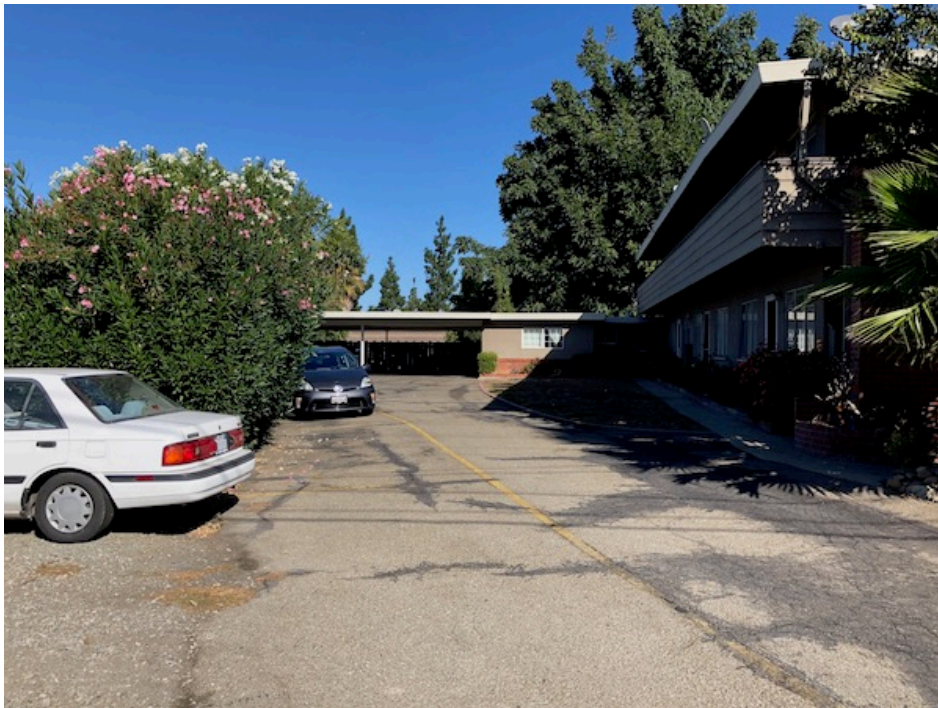
Photograph 5. View looking north at 2323 Moorpark from southeast corner of Site.
