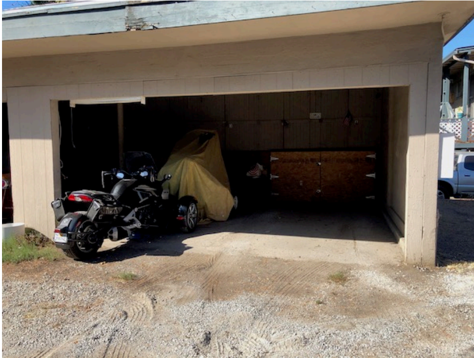
Photograph 30. Garage area along eastern side of apartments pictured in Photograph 29.
