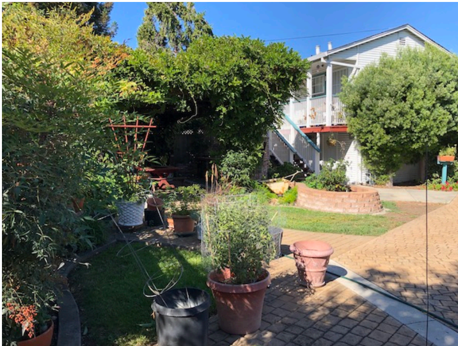
Photograph 35. Apartment building at 2379 Moorpark in center of Site.
