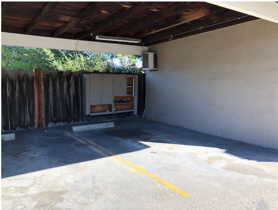
Photograph 7. Tenant storage cabinet within carport.
