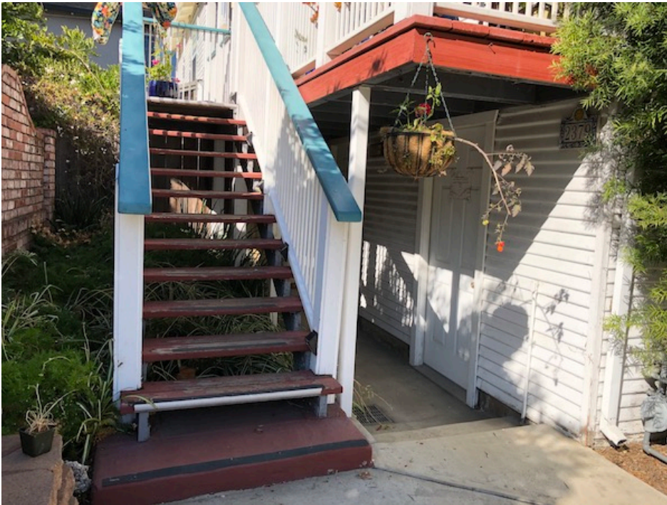
Photograph 37. Ground floor and stairway of apartment building at 2379 Moorpark.
