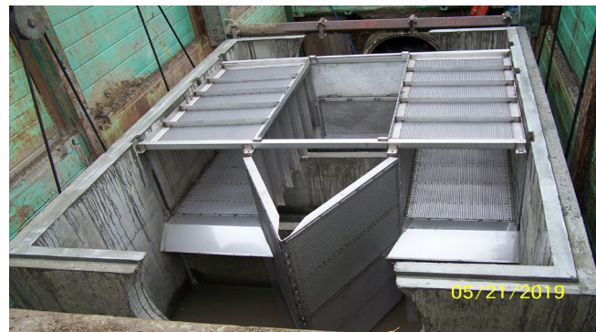
LTC device installation near Coyote Creek
