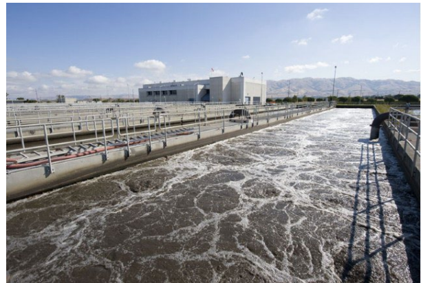
San José-Santa Clara Regional Wastewater Facility Aeration
