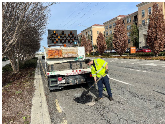
Pothole Repair
