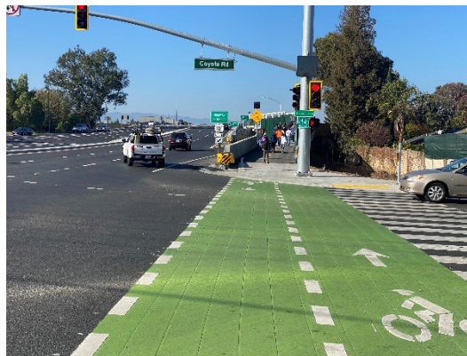
Bike Lane - intersection of Silver Creek Valley Rd, Coyote Rd & Hwy 101
