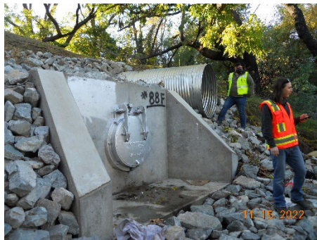
An outfall being rehabilitated
