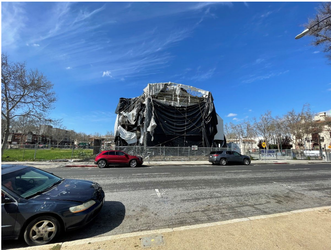
3/2023 Front of tarped building
