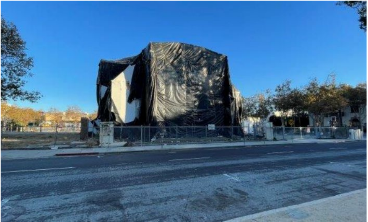
9/29/22 – Front of tarped building
