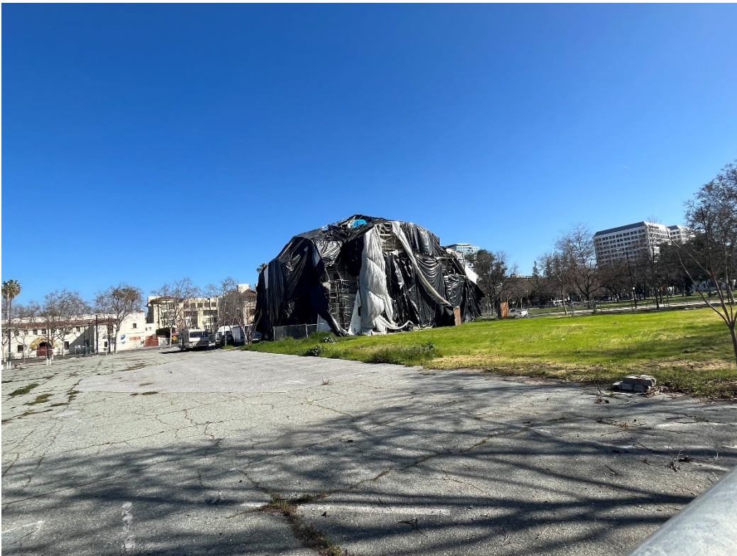
2/13/23 Rear of building
