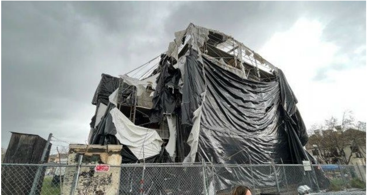
3/29/23 Front of tarped building
