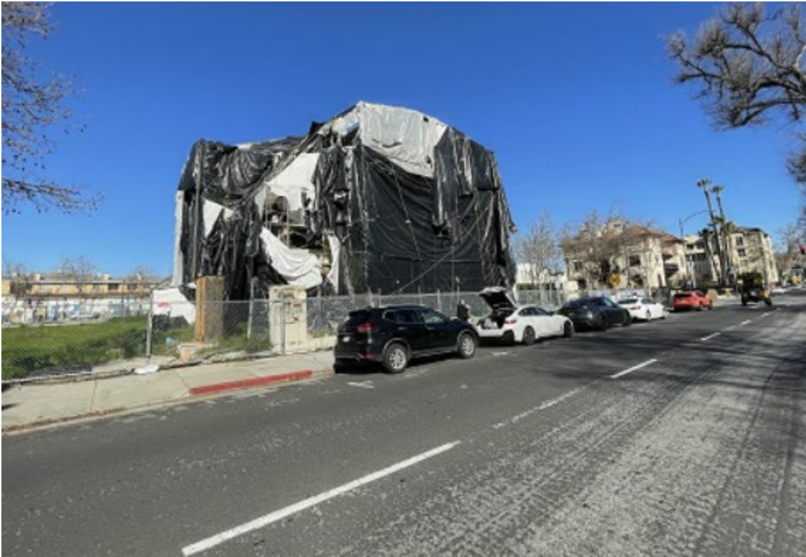
1/26/23 Front of tarped building
