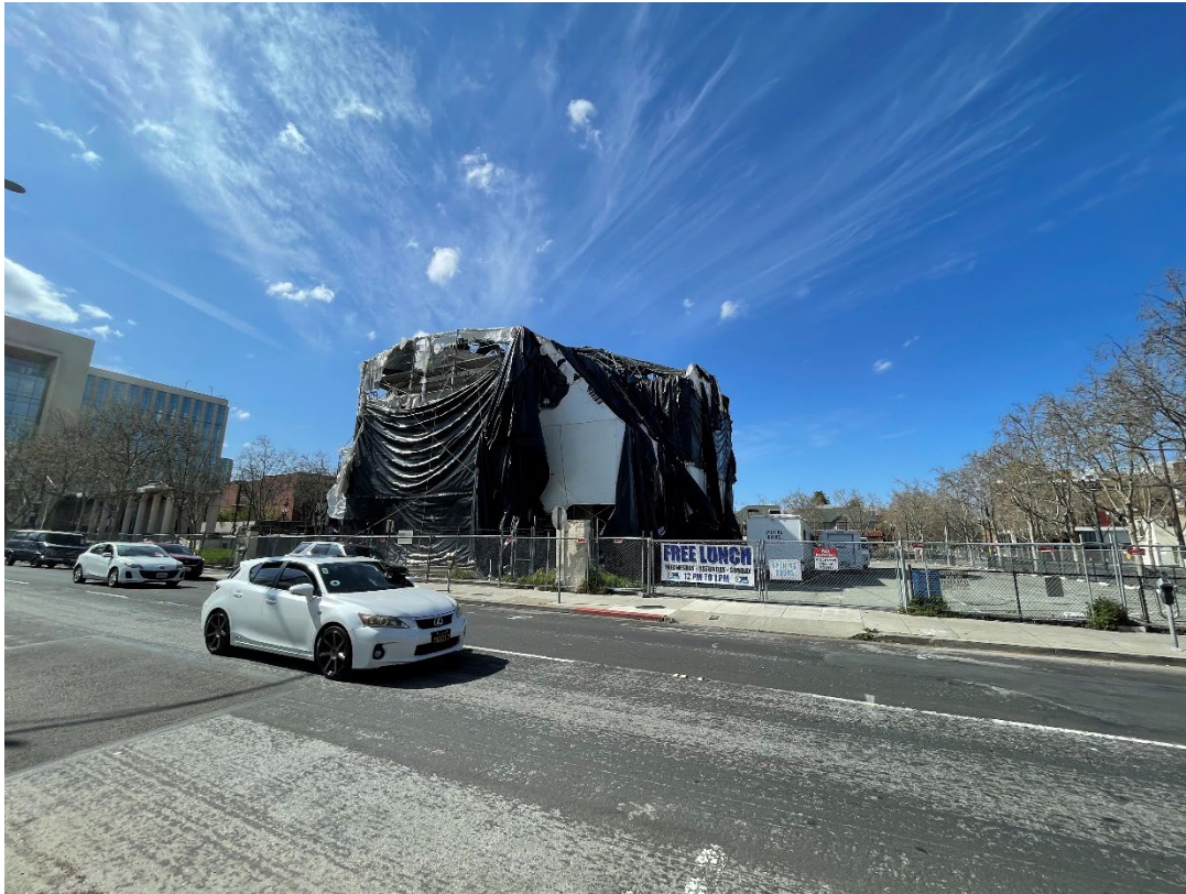
3/2023 Front of tarped building and food vending trucks in parking lot
