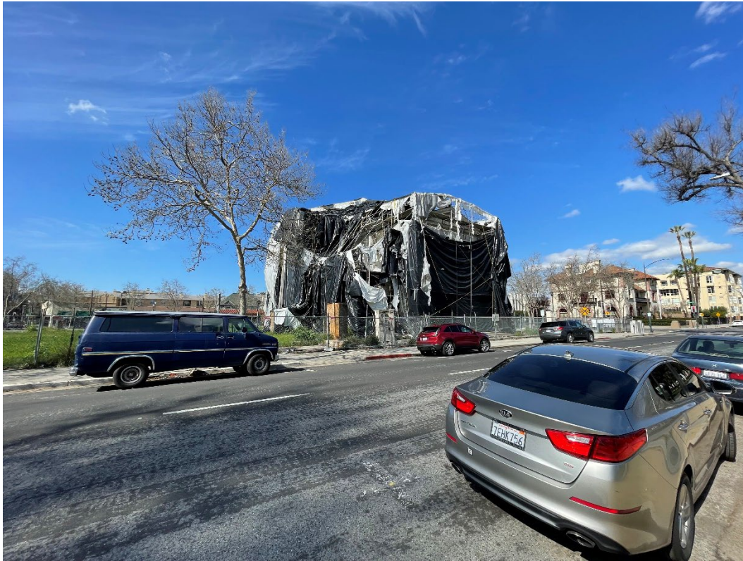
3/2023 Front of tarped building
