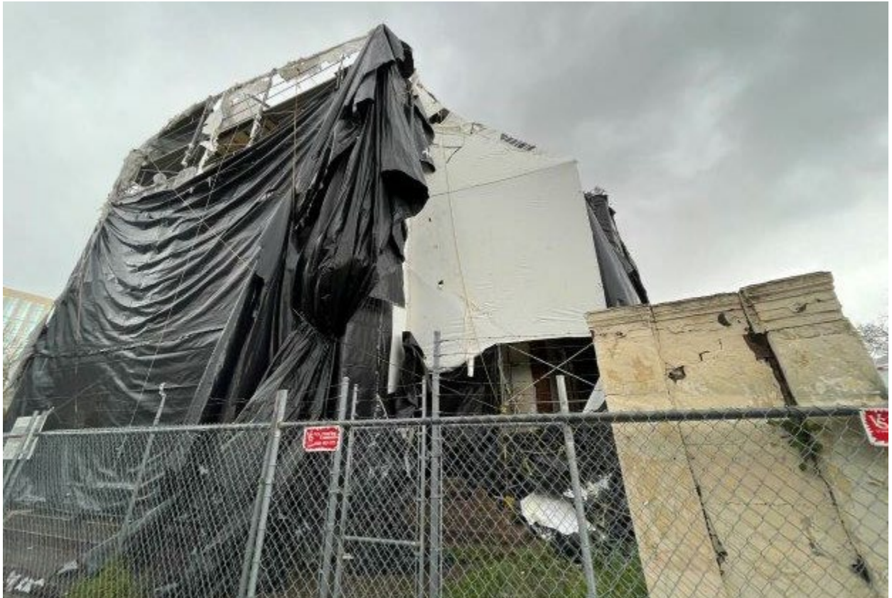
3/29/23 Front of tarped building
