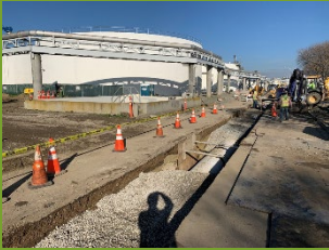
Storm Drain Pipe Replacement
