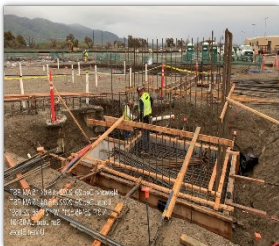
Rebar installation at Dewatering building
