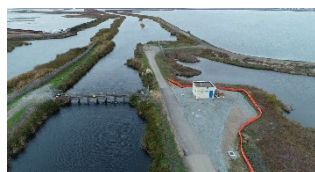
The weir structure and Sulfur Dioxide building at the outfall channel.
