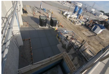
Transformer pads and installation.
