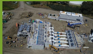
Aerial view of the new Raw Sewage Pump Station and Grit Facility.
