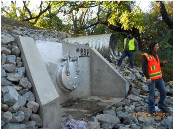
An outfall being rehabilitated
