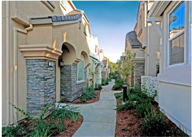
Shared walkways like this one in Willow Glen are one of many site design low impact development (LID) techniques used in the City
