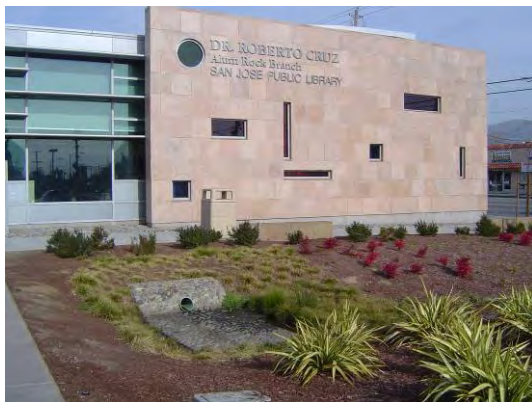
Alum Rock Library extended detention basin, a stormwater treatment control measure
