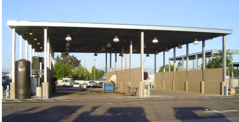
Bermed and covered vehicle wash pad at the Central Service Yard.
