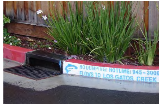
Storm drain inlet stenciled with the name of the nearest creek and the City's stormwater dumping complaint number
