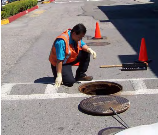
ESD Watershed Enforcement Inspector observing a grease interceptor at a San José mall
