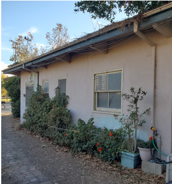
Figure 16. East elevation of garage and brick pavers, looking southwest.
