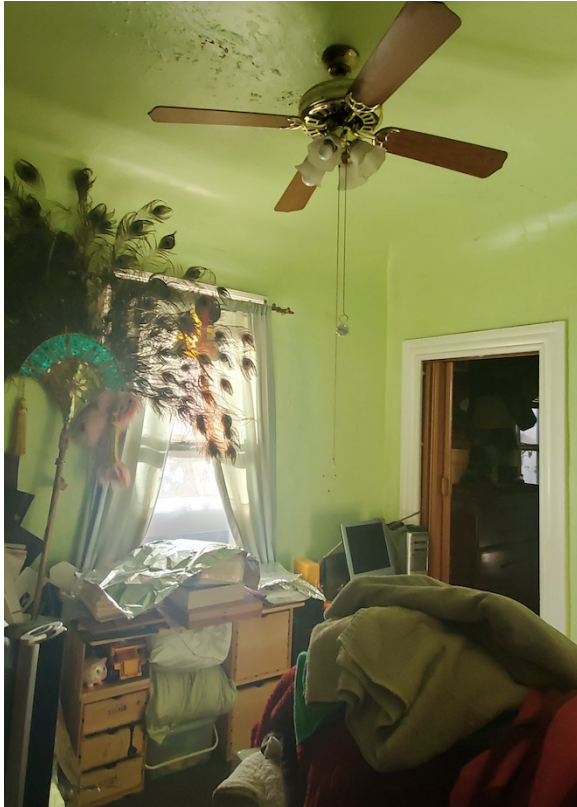
Figure 20. Bedroom 1 with light green painted plaster walls, window and classical door molding.
