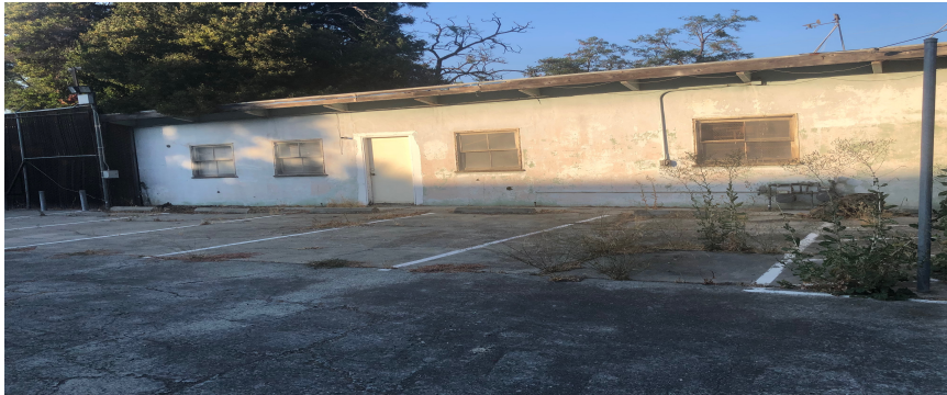
Figure 14. West elevation of garage building looking east.
