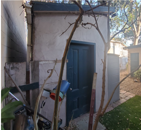
Figure 7. Shed between garage and house, looking east.
