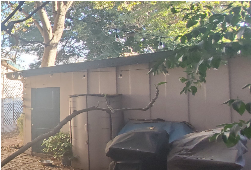
Figure 15. North elevation of garage looking southeast.
