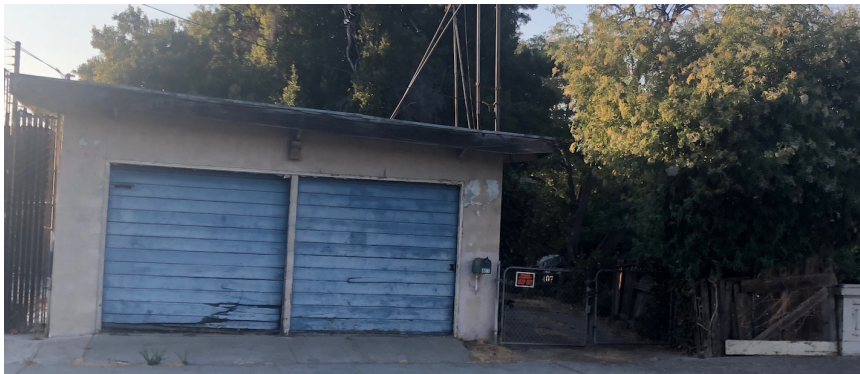
Figure 4. View of 407 along W. St. John Street, facing north (GA).
