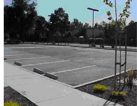
Porous-paved parking lot: a stormwater site design and treatment control measure
