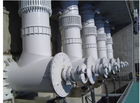
Pumps at the Rincon II Pump Station
