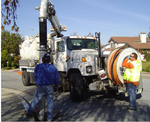
Department of Transportation Vector crew cleaning out a storm drain inlet
