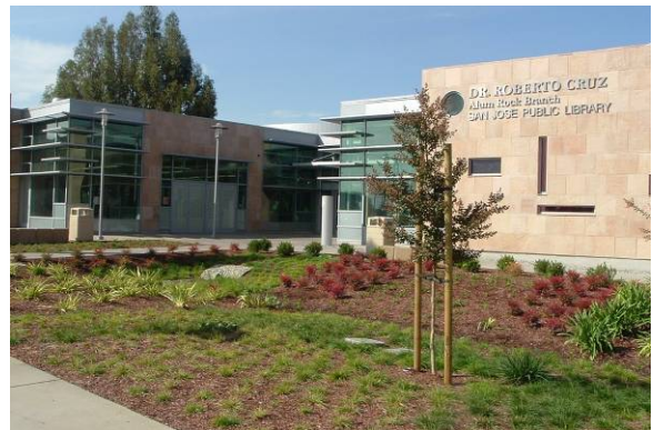
Alum Rock Library detention pond, a stormwater treatment measure
