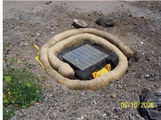
Proper storm drain protection during construction prevents construction debris and sediment from entering the storm drain
